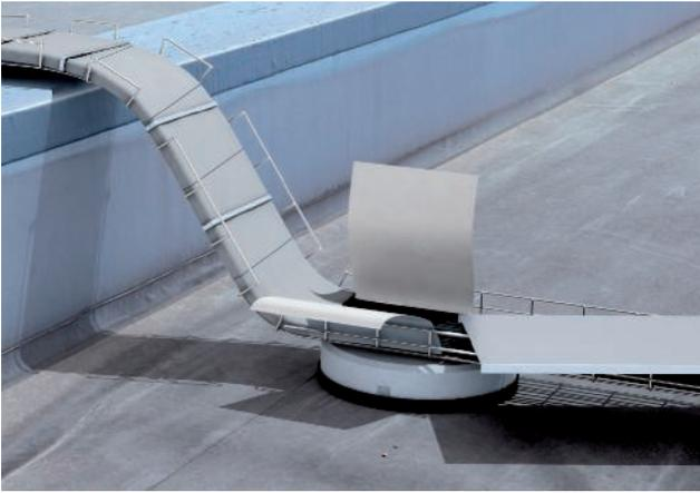
Bandaged cables routed over a firewall
