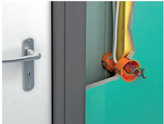
Approved installation of opposing standard cavity wall sockets besides doors without fire resistance.
